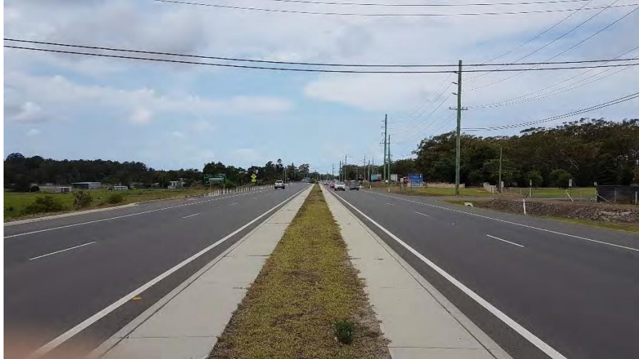
Plate 12-1: Nelson Bay Road looking east in the vicinity of the subject site.
