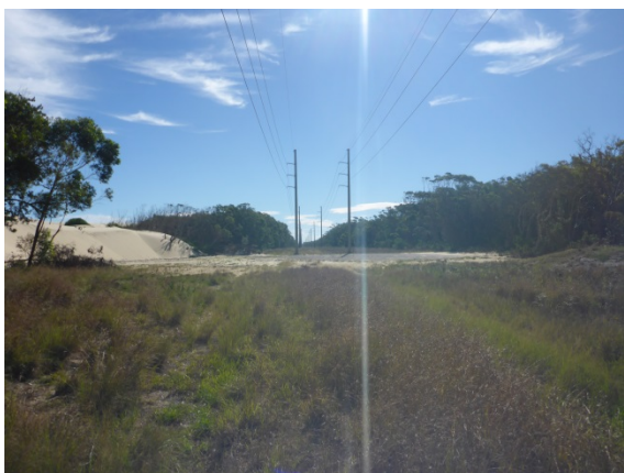
Photograph 3 Looking west along the electricity transmission easement from the eastern site boundary.
