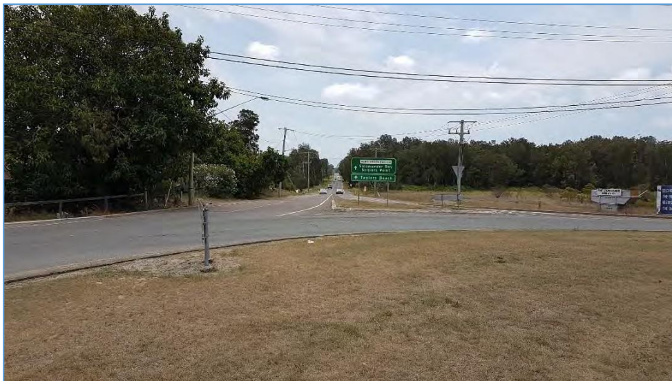
Plate 12-9: Port Stephens Drive looking north from Nelson Bay Road Roundabout
