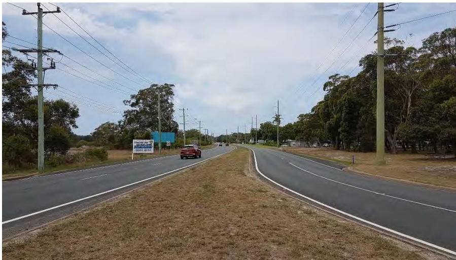
Plate 12-2: Nelson Bay Road looking east from Nelson Bay Road / Port Stephens Drive Roundabout
