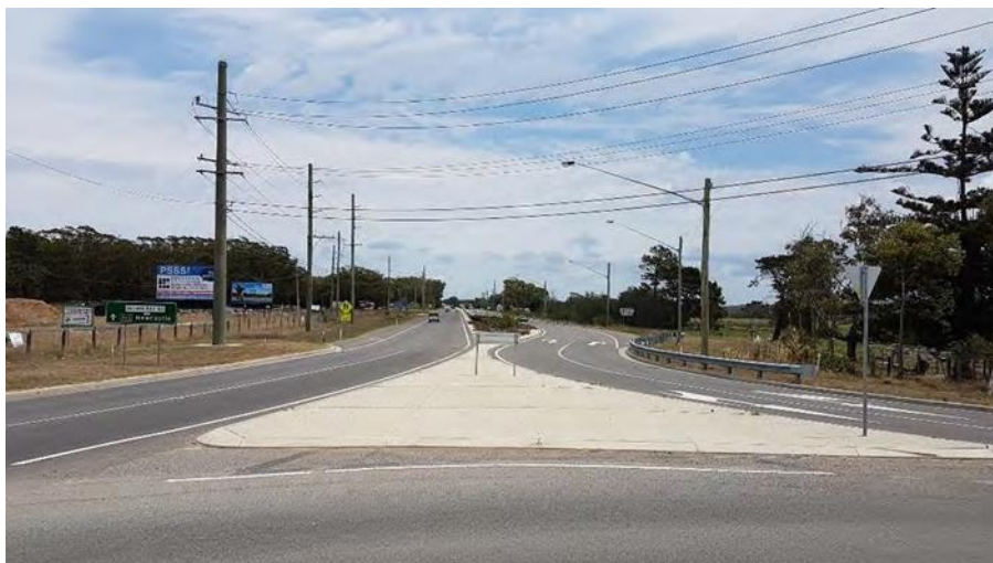
Plate 12-3: Nelson Bay Road looking west from Nelson Bay Road / Port Stephens Drive Roundabout.
