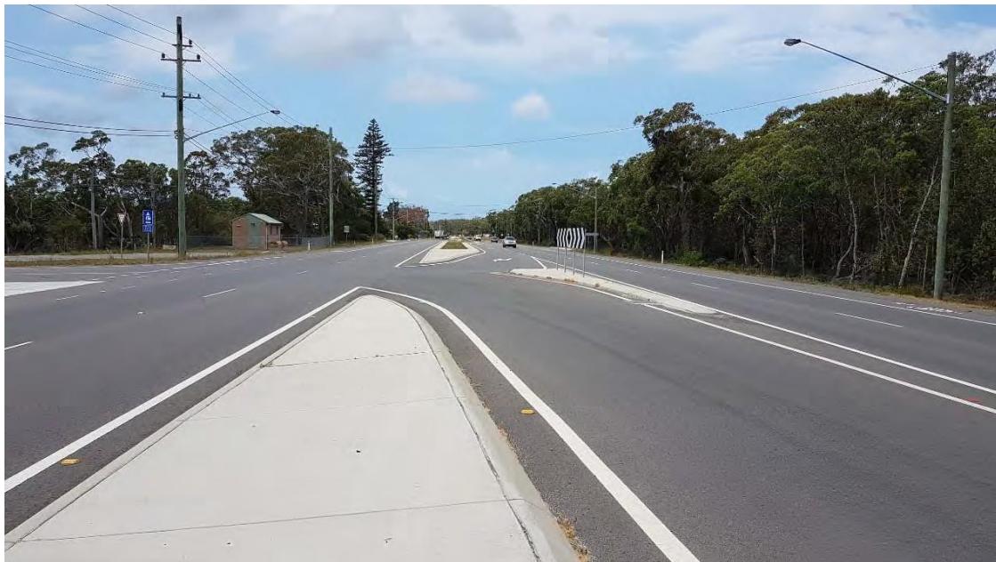
Plate 12-5: Seagull intersection allowing right turn movements at Nelson Bay Road / Trotter Road (looking east)
