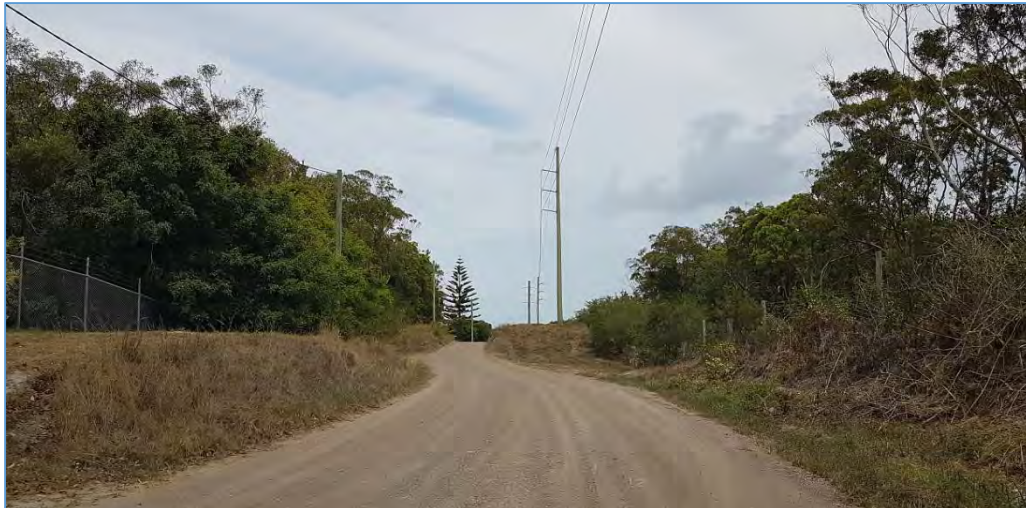
Photo 13 – Jessie Road looking south
