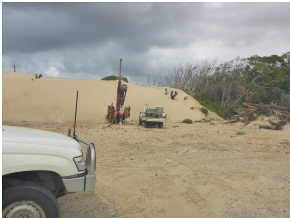
Photograph 11 Borehole drilling at the location of BH6/PZ2.
